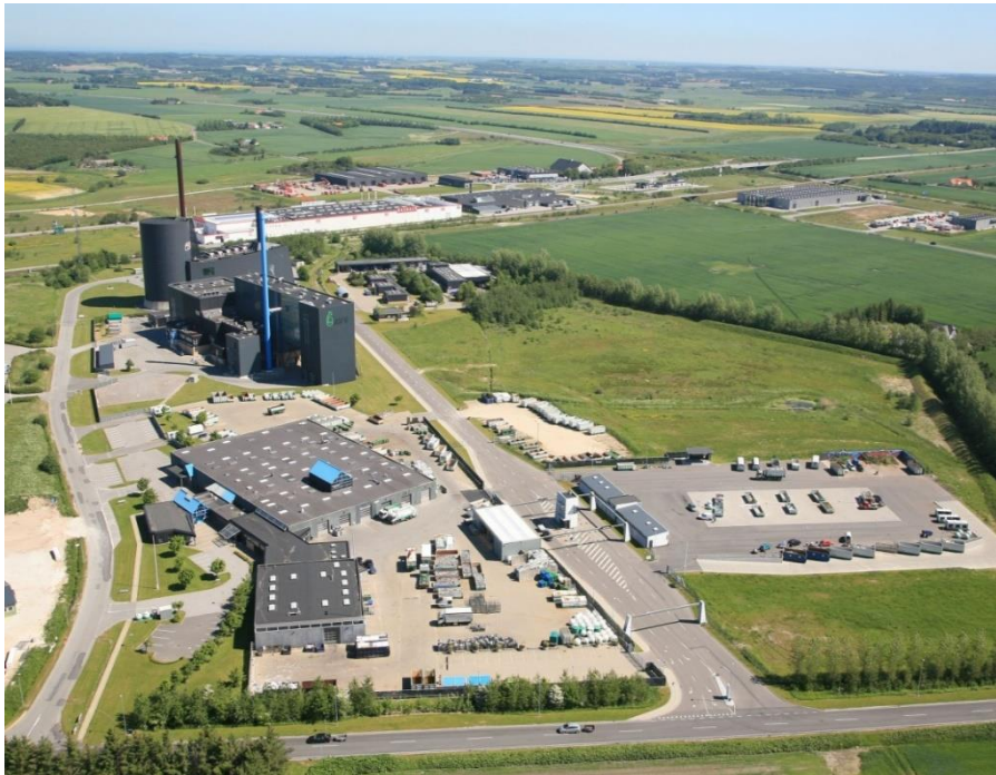
Figure 4.1 AVVs current facilities were established in 1988. In the back is the incineration plant. In the front is the administration building incl. the reuse shop and halls for preparing waste for reuse and recycling. To the right is the largest of AVVs recycling centers.
