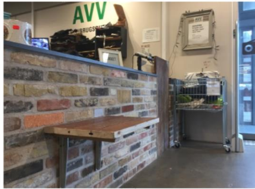
Figure 4.12 The counter in AVVs reuse shop is built of old bricks
